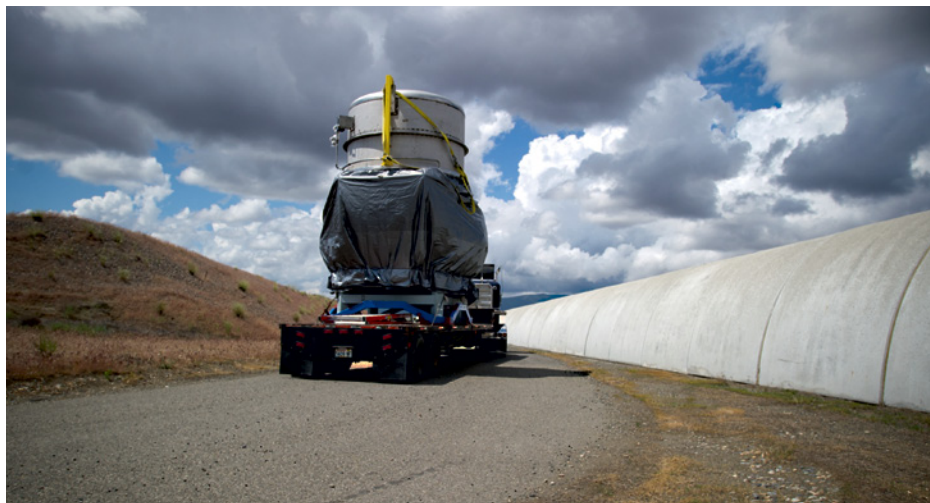
The 10 tonne BSC6 chamber departs the Y mid-station at LIGO Hanford, destined for the end station building. The chamber was relocated to transition the H2 interferometer from its Initial LIGO 2 km length to that of Advanced LIGO, 4 km. With the advent of LIGO India, the H2 chambers now remain empty, an opportunity for future interferometer configurations.
