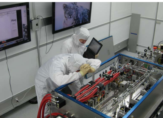
Top: Peter, Oliver and Mike lifting the 300 kg High Power Oscillator onto the laser table at L1. This was the first thing brought inside the new build room and the first item on the cleaned PSL table. At that time the room was not yet operated as clean room.
