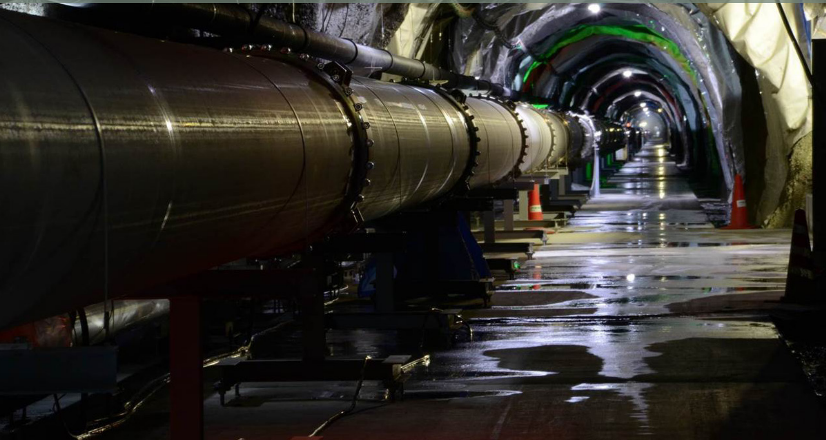
▲ KAGRA's Y-arm under construction
