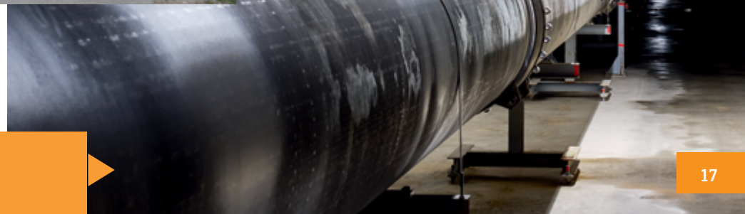
KAGRA 3km arm cavity in the underground tunnel.
